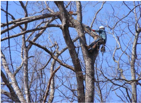
Removal of hanging tree limbs was a major part of ice storm recovery efforts.
