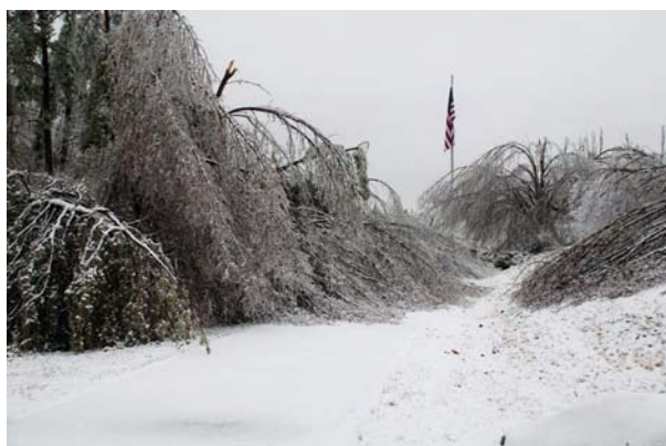
Entrance to LBL's Administrative Office after the ice storm.
